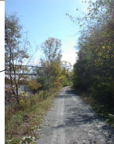
Weldon Creek Bridge
